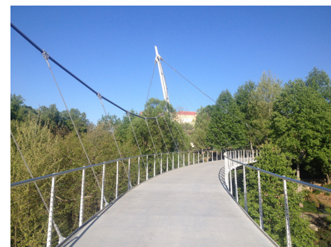
Liberty Bridge in Greenville, SC rises to the level of civic art and provides a key linkage in that town's greenway network.
