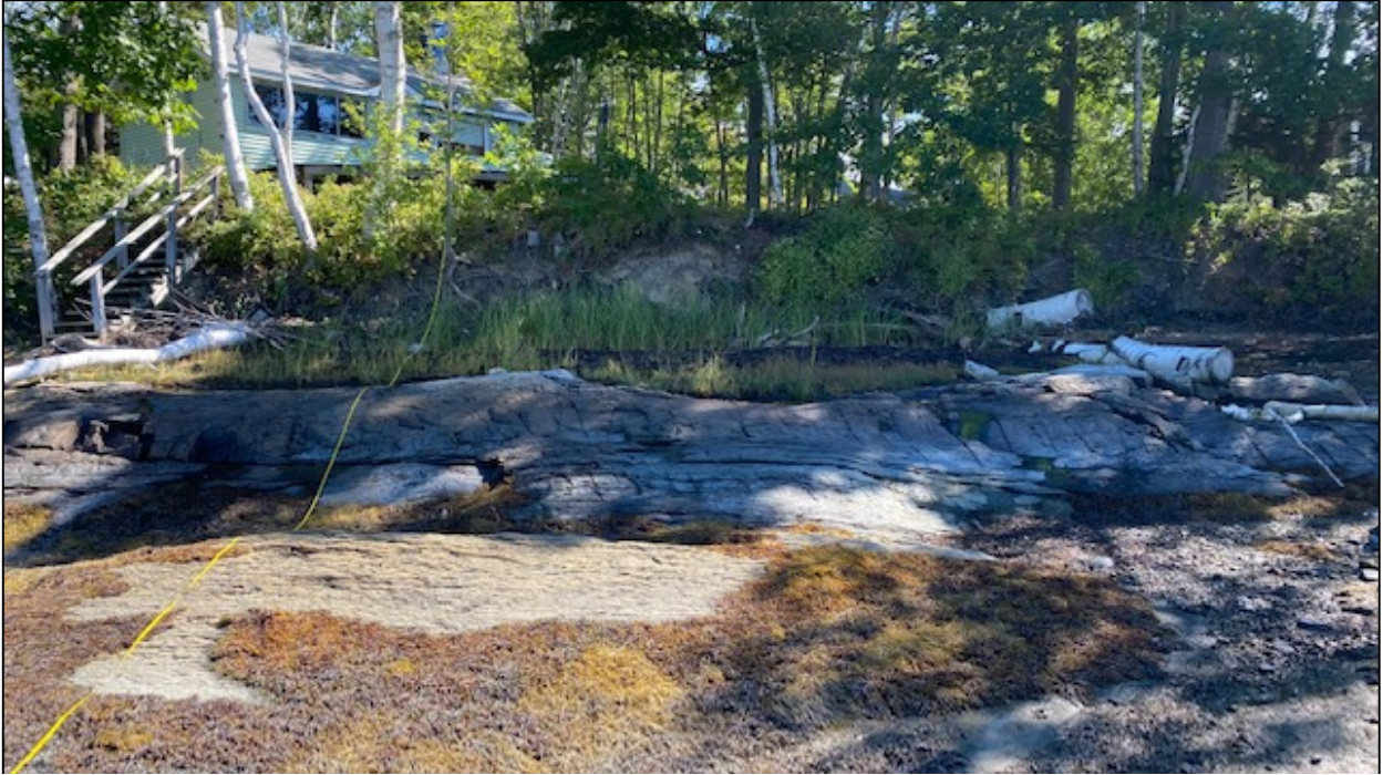
Photograph Seven. View of existing stairs that will be removed. Tape measure shows location of proposed pier. Photographer: Tim Forrester, Atlantic Environmental, LLC Date: September 16, 2021.
