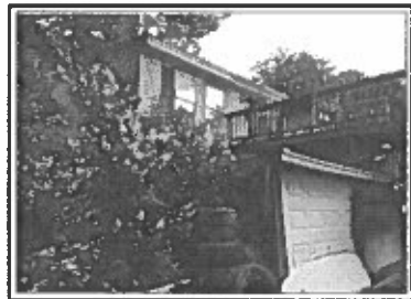
Back of Garage and Inlaw 2nd View
