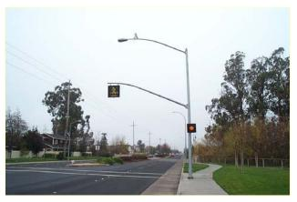
• In-pavement flashers – Installed with a flashing sign at the crosswalk and advanced flashing sign (such as shown on the right, on El Dorado Street in downtown Stockton). Installed with audible warning, advance signs, rumble strips, and single sided indication, per CTCDC requirements.
