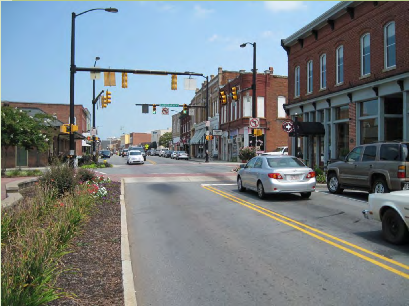
Buried Utility Lines/Poles
