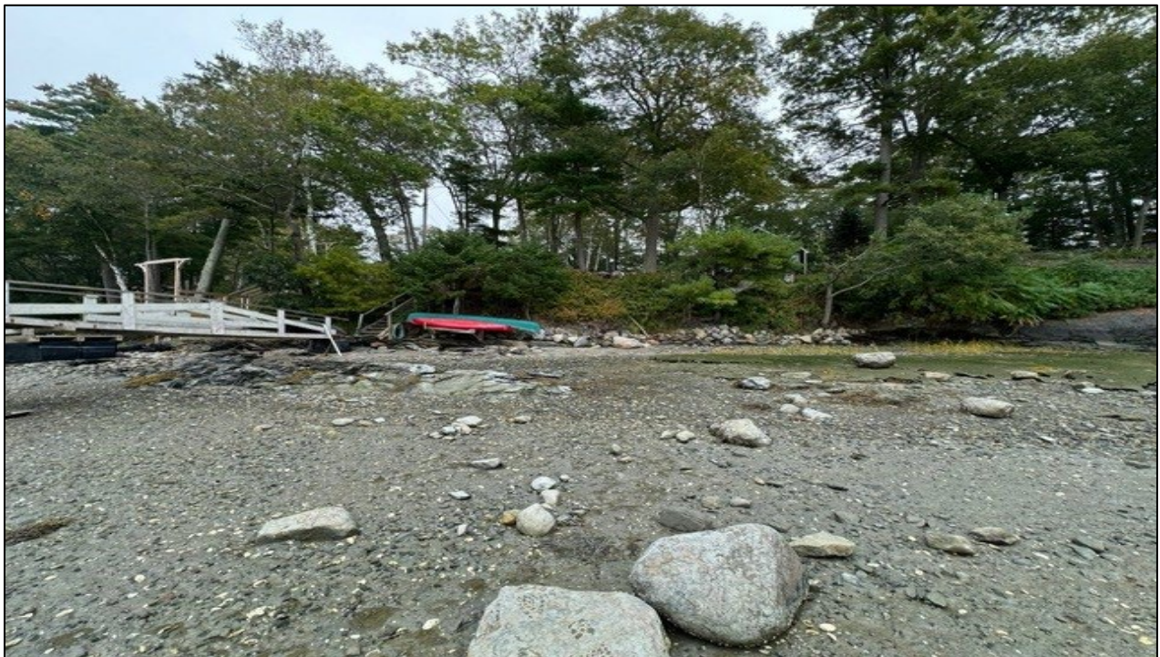
Photograph Six. Facing easterly. View of intertidal zone, eroding shoreline to be stabilized and existing structure to be removed.
