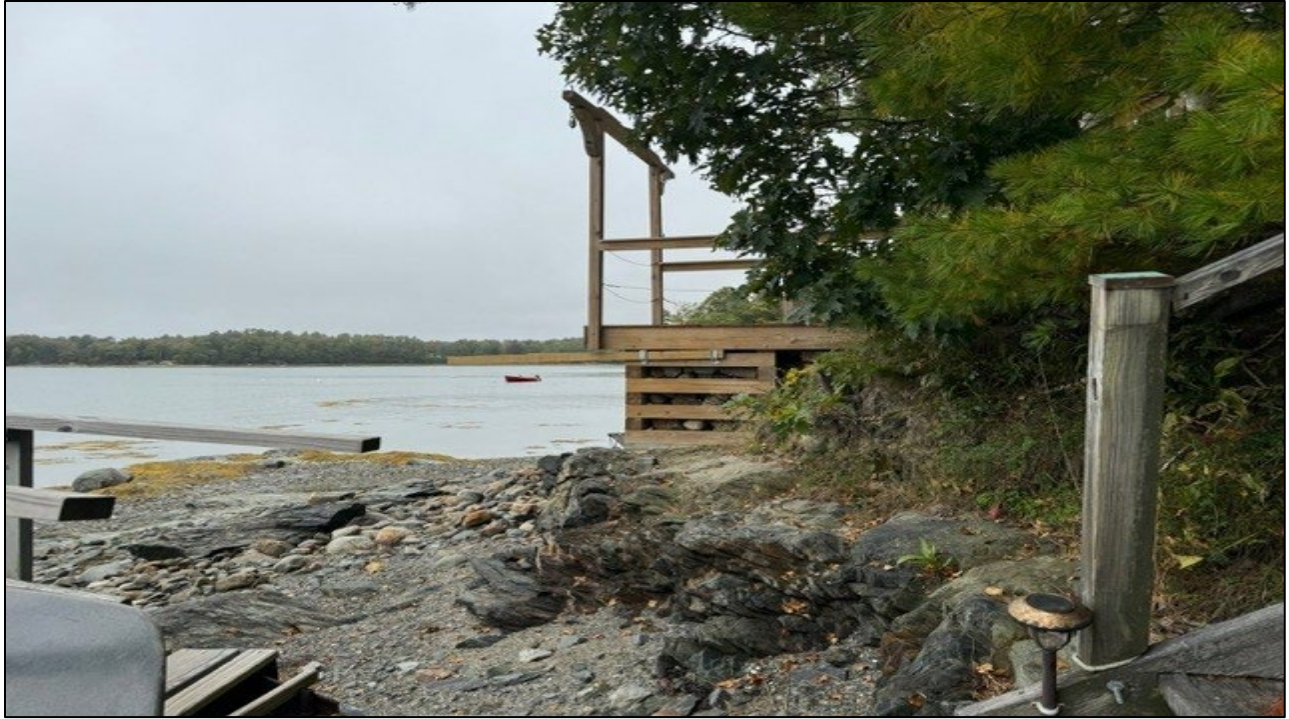
Photograph Five. Facing northerly. View of existing structure in the foreground to be removed. View of abutting structure in the background.
