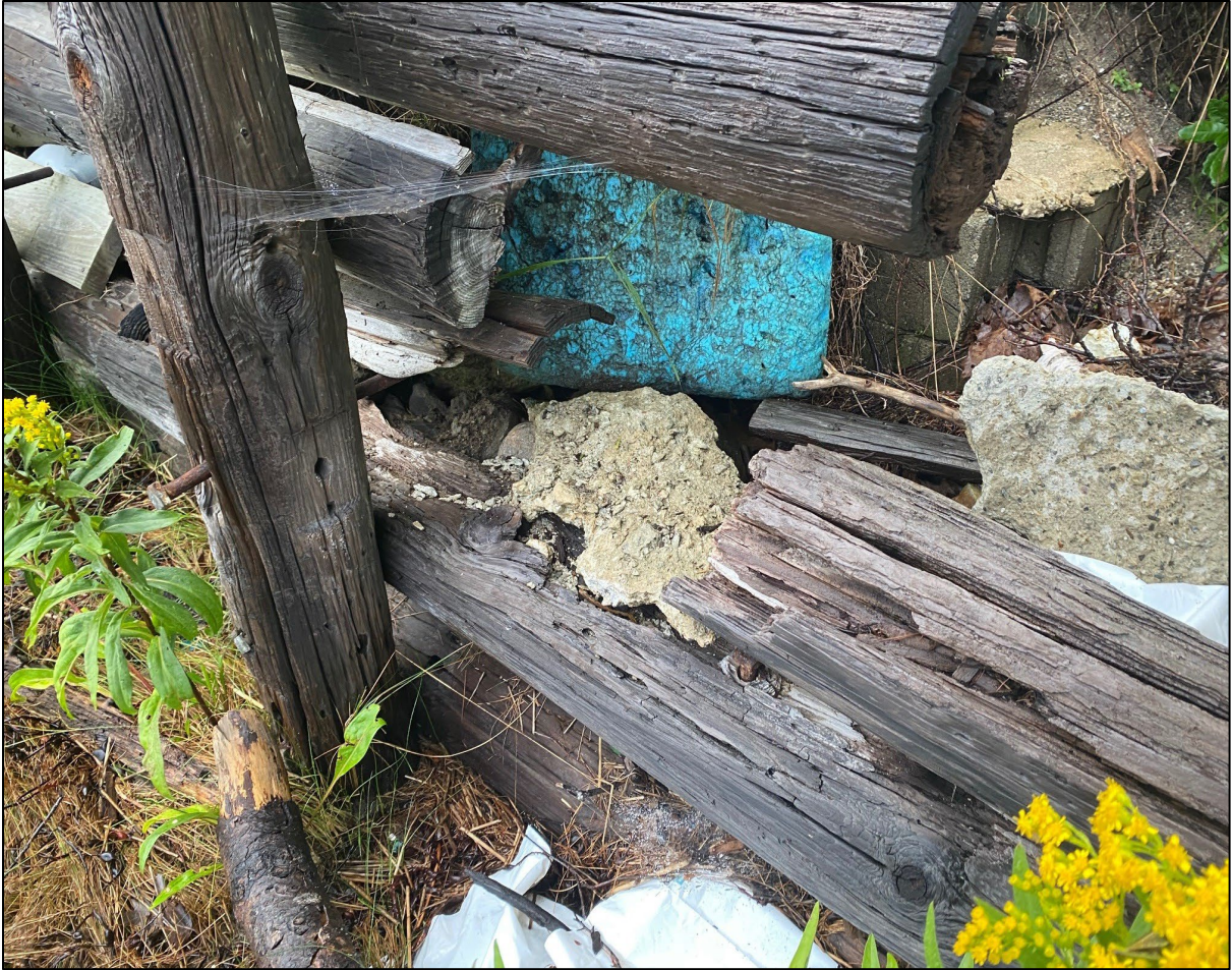
Photograph Seven. Additional view of timber retaining wall.
