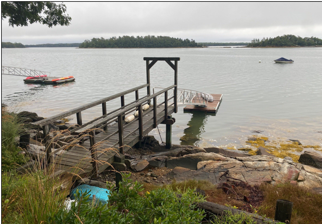
Photograph Two. View of existing dock from upland.
