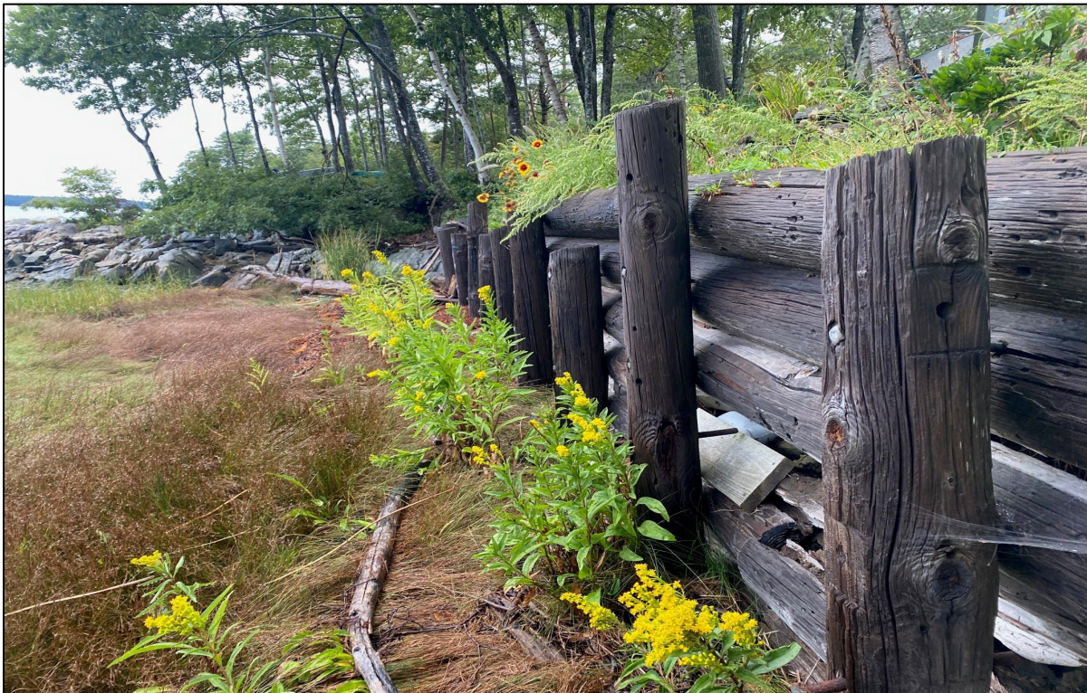
Photograph Six. Additional view of timber retaining wall and intertidal zone.
