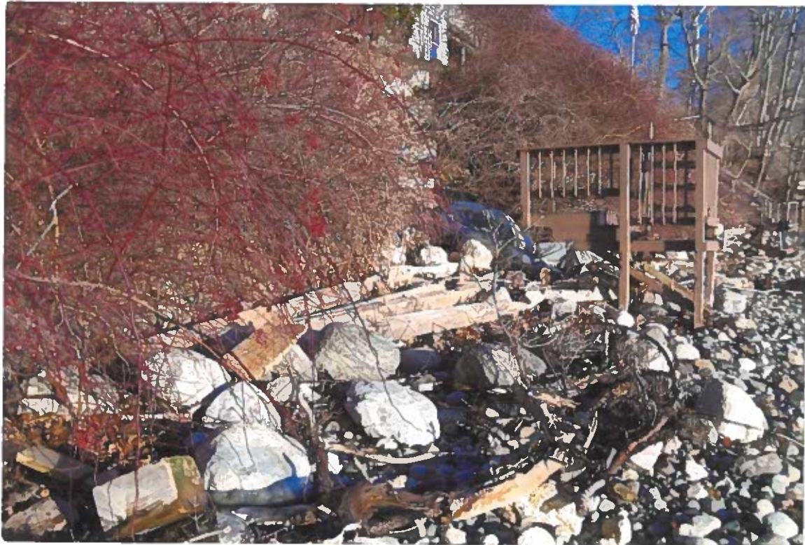
Retaining wall and landing post 2022 storms
