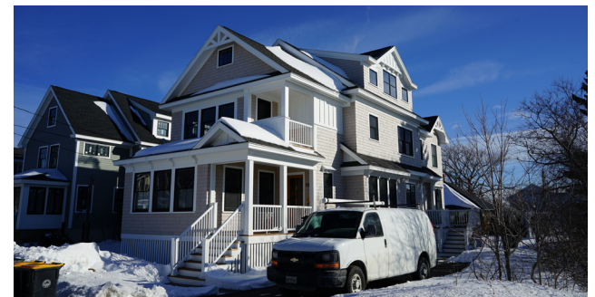
A house built under the new zoning.
