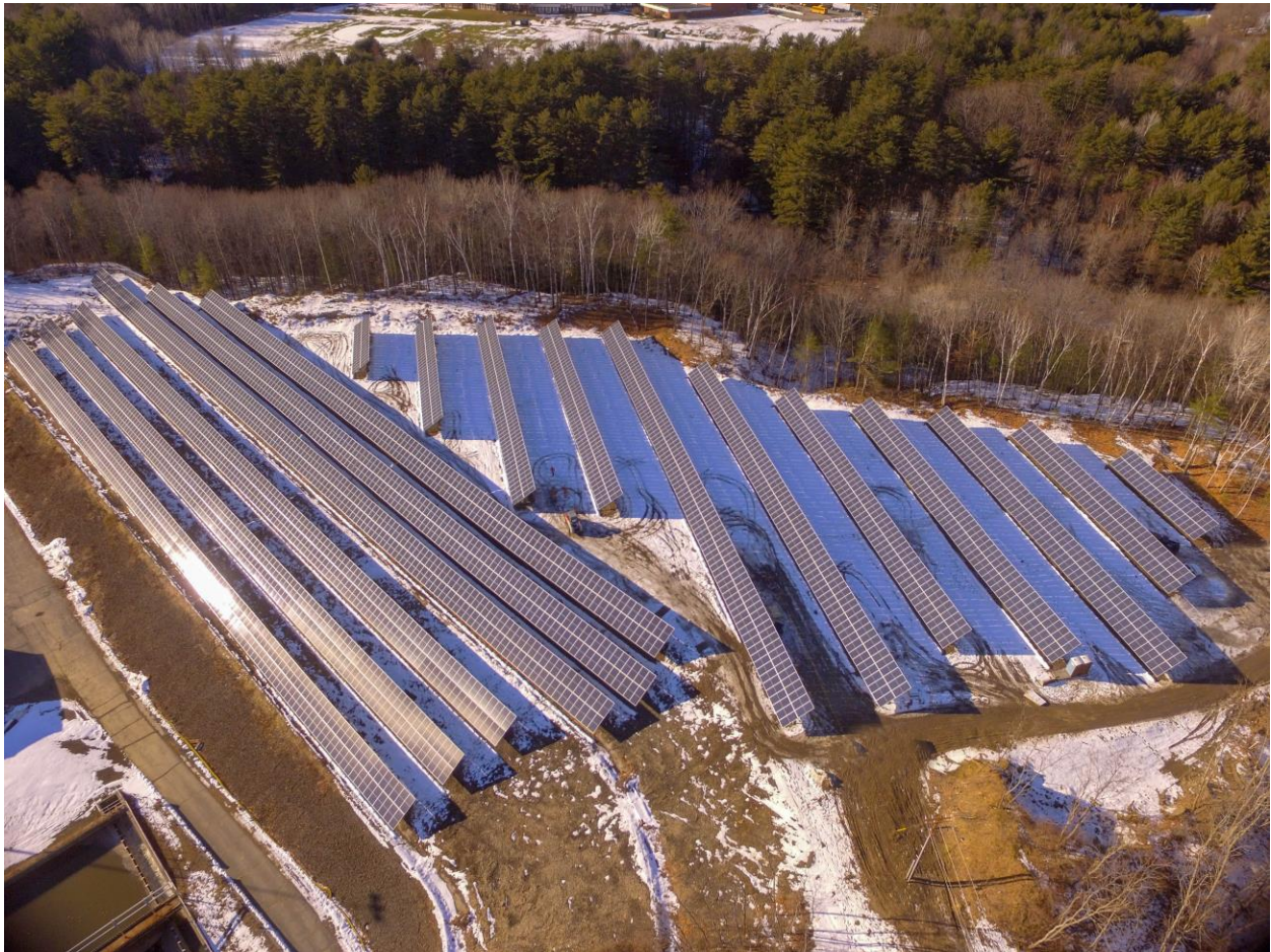
Figure 1. A 968.76 kW solar array installed for the Kennebec Sanitary Treatment District in Waterville, Maine, by ReVision Energy.
