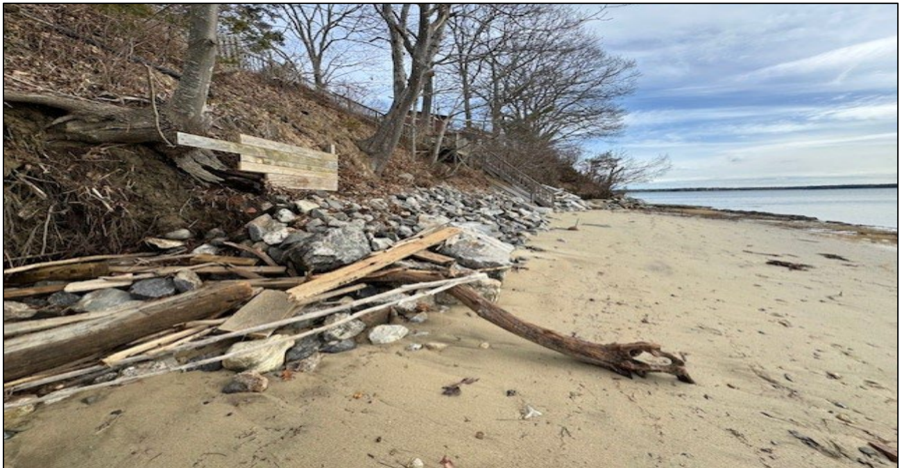
Photograph Four. Facing northeasterly - additional view of shoreline showing existing conditions.
