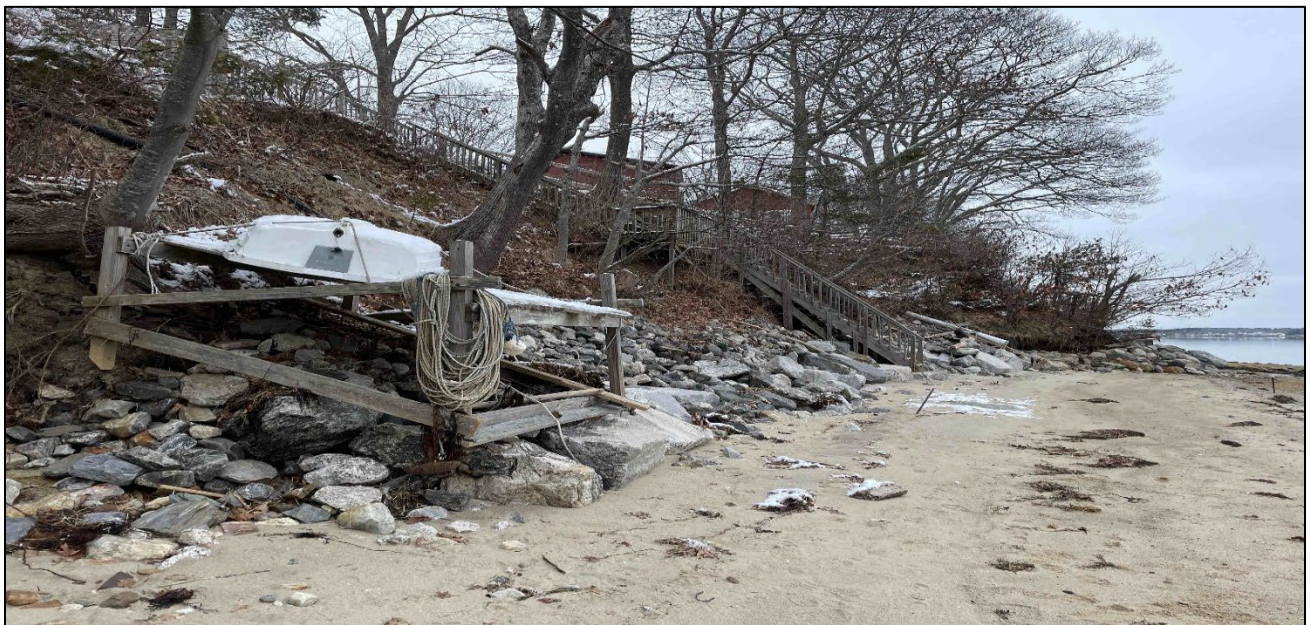
Photograph Two. Facing northeast. View of area of shoreline where small riprap has washed down slope.
