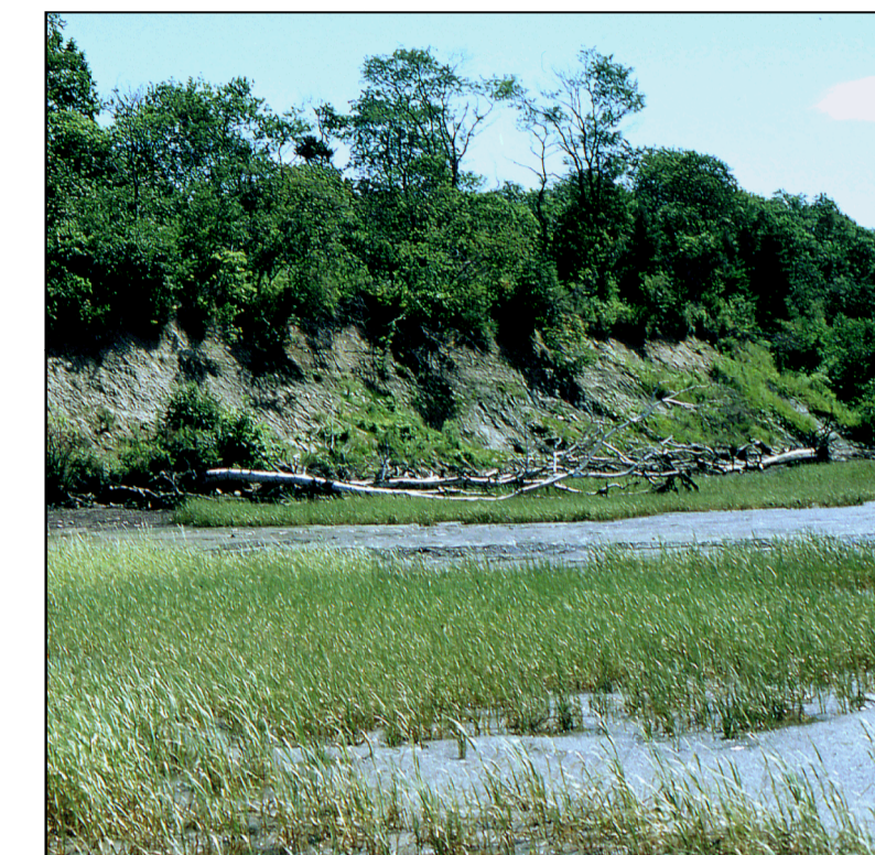
Highly unstable bluff with an unvegetated bluff face and a salt marsh shoreline. Sediments on the bluff face are exposed and fallen tree trunks lie at the base of the bluff. A salt marsh has recently formed on the tidal flat, partly on the top of an old landslide deposit.
