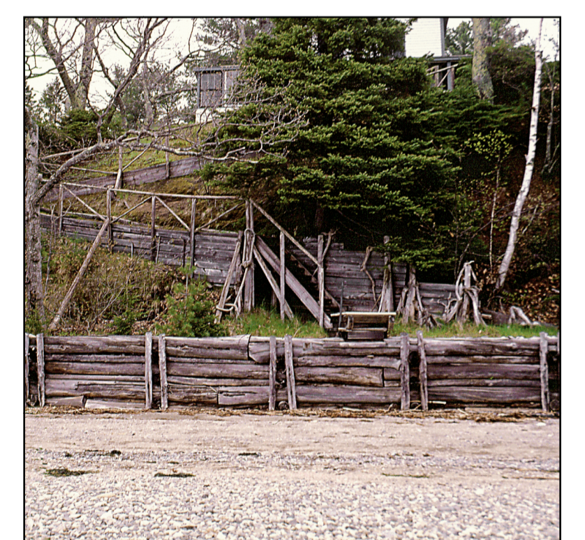
Stable bluff with a vegetated bluff face and an armored shoreline. The bluff face is fully vegetated and supports a mature stand of trees with vertical trunks. The presence of a wooden bulkhead suggests that erosion has occurred in the past.
