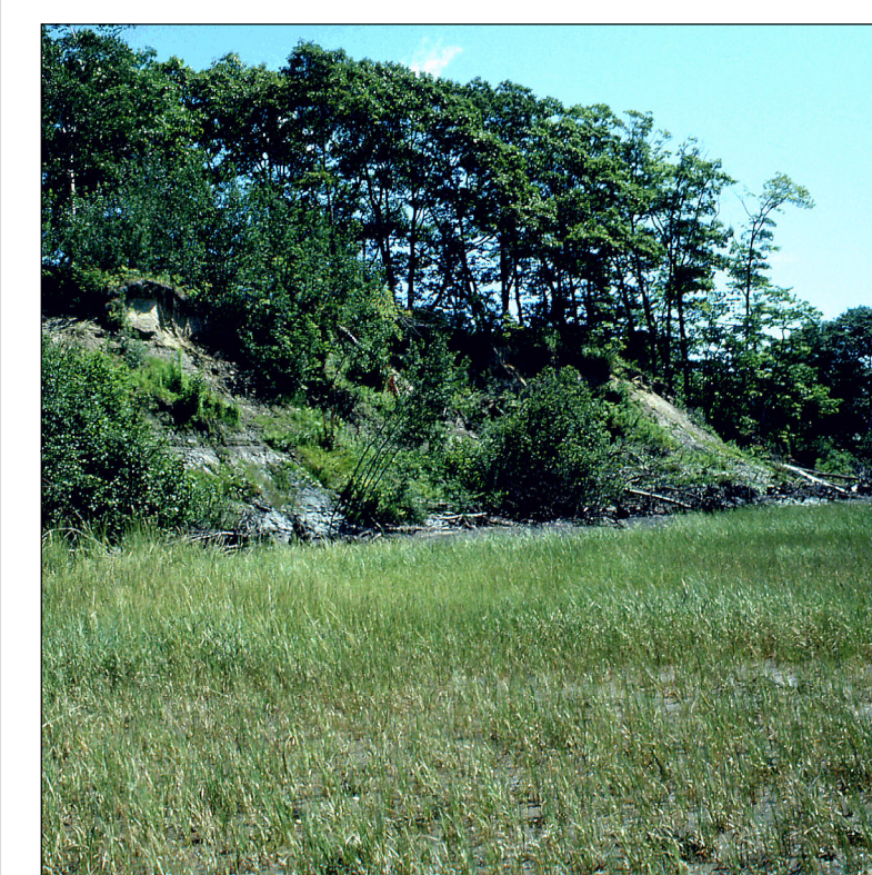
Unstable bluff with a partially vegetated bluff face and a salt marsh shoreline. This bluff, protected by a salt marsh, remains unstable. There are small bushes on the bluff as well as small non-vegetated areas that indicate continuing bluff retreat.
