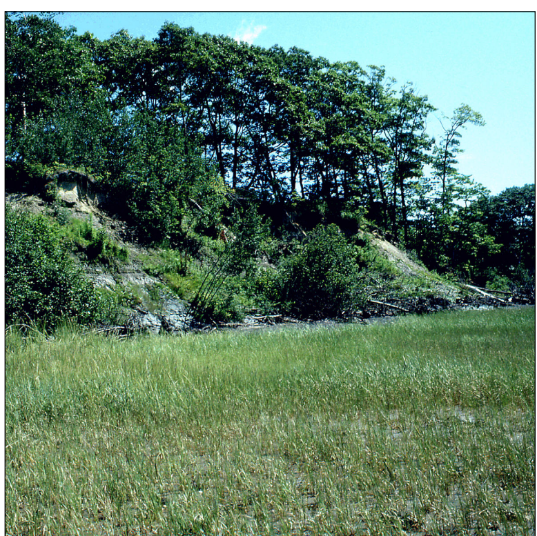
Unstable bluff with a partially vegetated bluff face and a salt marsh shoreline. This armored bluff is eroding despite an effort to shore it up with riprap, or loosely piled stone blocks. Maintenance at this site could improve bluff stability.
