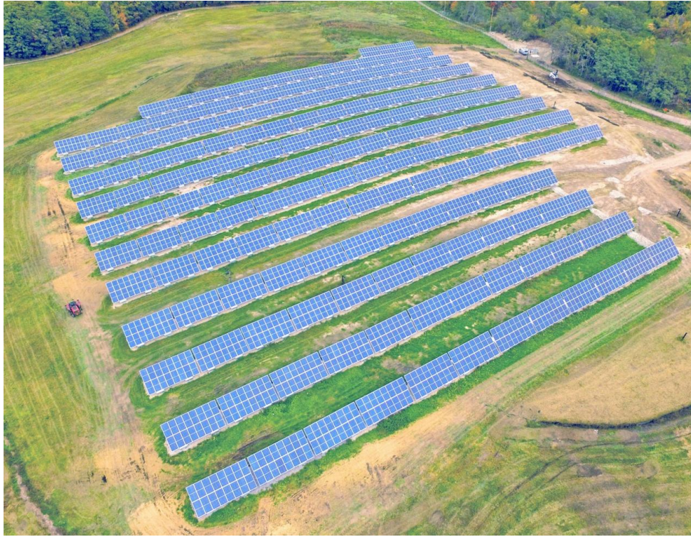
City of Portland, ME 660 Kilowatts
