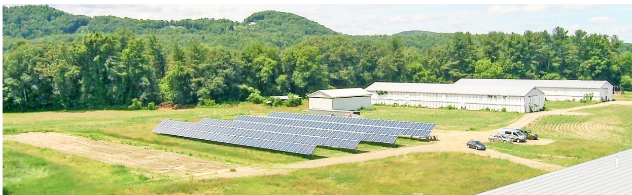
Chamberlain Machine - Walpole, NH 132 Kilowatts (400 solar panels)
