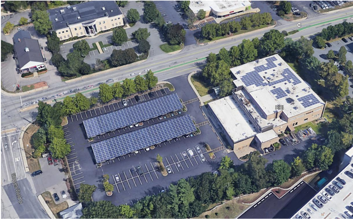
REI Store, Framingham, MA 210 Kilowatts (parking lot & roof)
