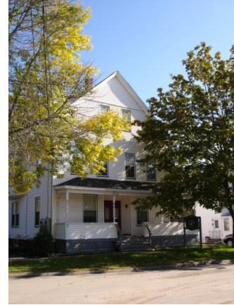
Front Porch facing street.
