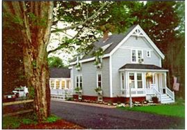
Horizontal siding with trim at openings and along building edges.
