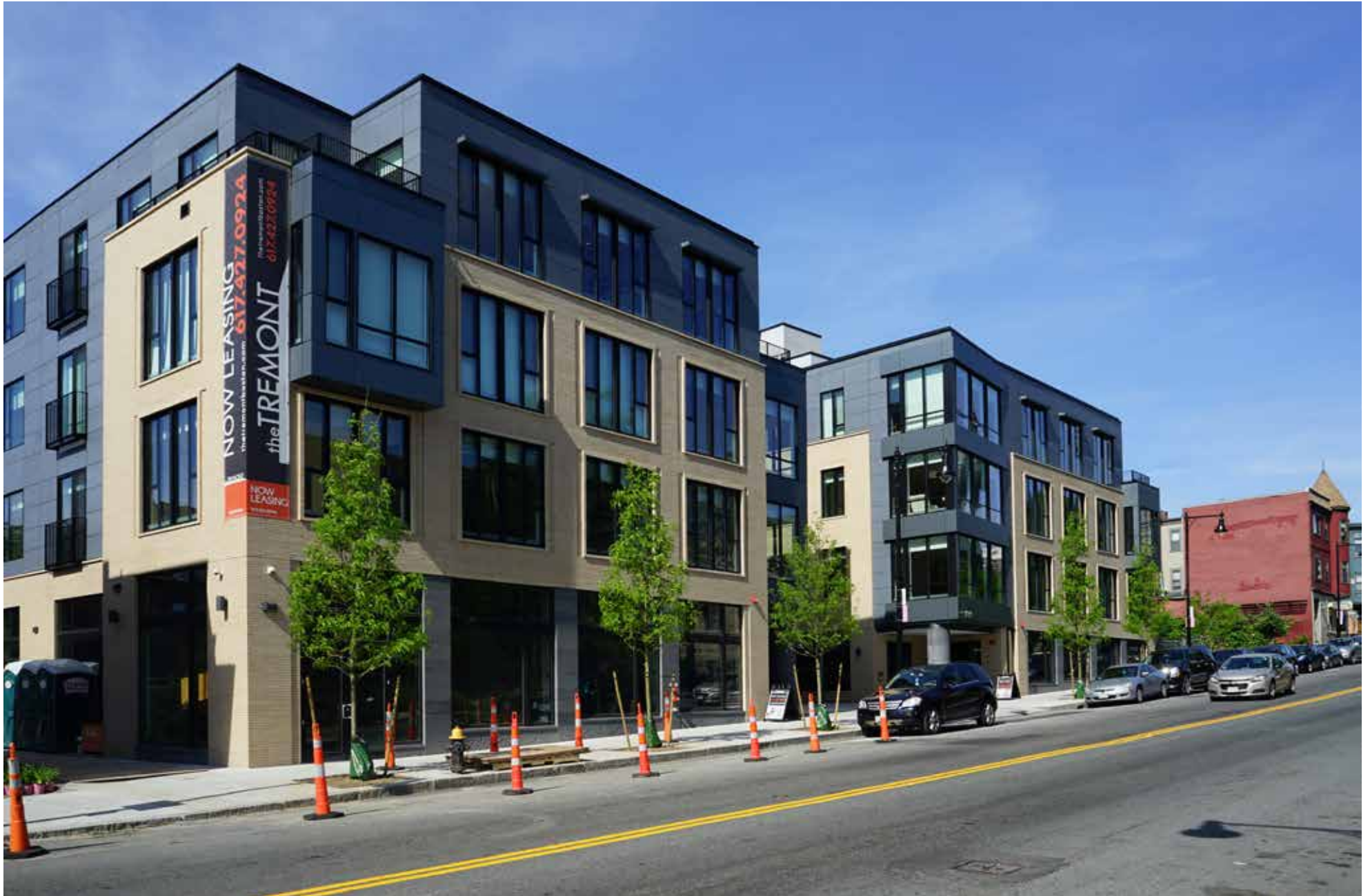
The Tremont looking southwest.
