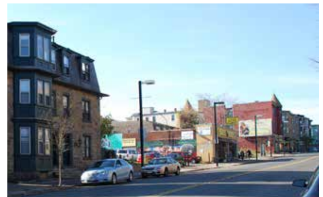
View of the site prior to construction.
