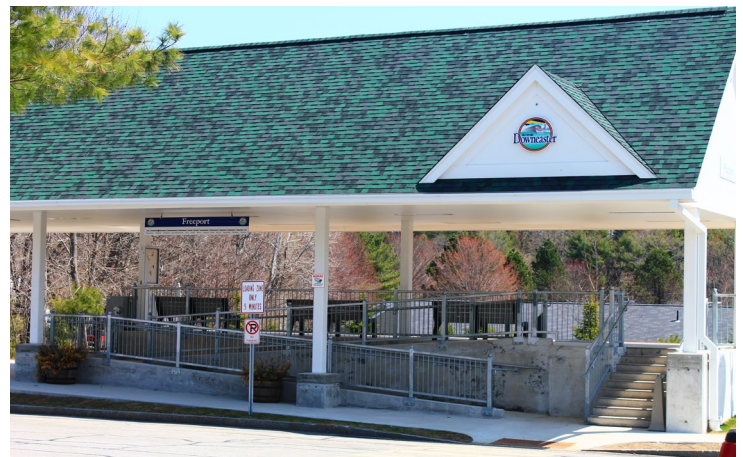
Train Station Platform Photo Courtesy Town Staff
