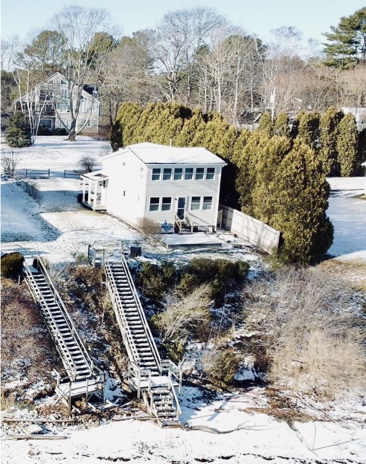
Photograph Two. Facing Northwest - view of eroding slope.
