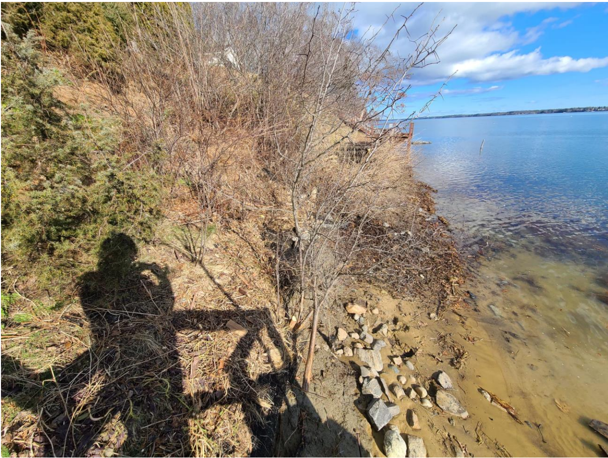
Photograph Four: Facing North, view of the exposed soil and eroded embankment.
