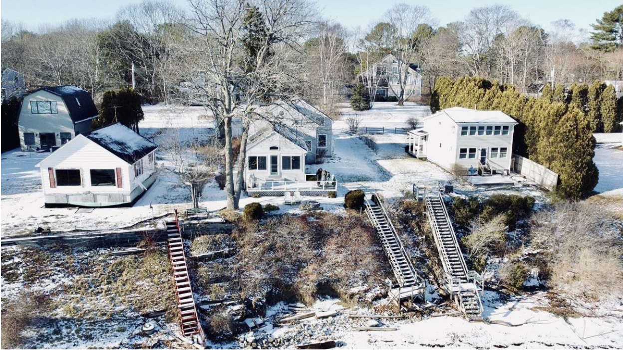
Photograph Five: Drone Shot Facing Northwest:
