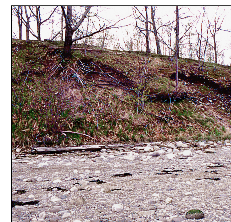
Unstable bluff with a partially vegetated bluff face and a beach/gravel flat shoreline. Slump scars on the bluff face expose sand, gravel, and roots. Fine sediments are removed by waves and currents, leaving gravel to form a beach at the base of the bluff.
