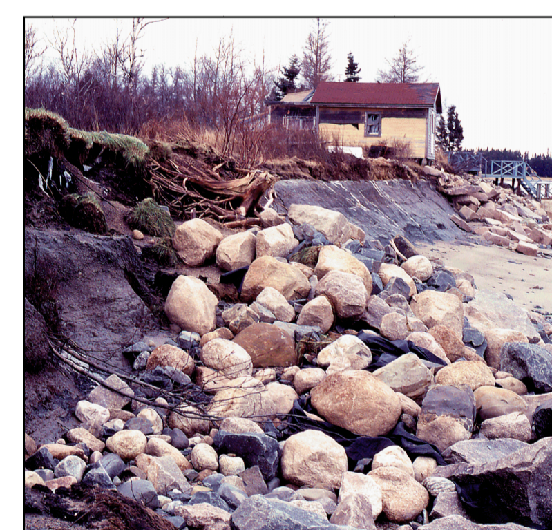
Highly unstable bluff with an unvegetated bluff face and an armored shoreline. This armored bluff is eroding despite an effort to shore it up with riprap, or loosely piled stone blocks. Maintenance at this site could improve bluff stability.
