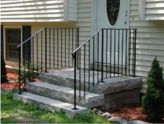
Precast Concrete steps with powder coated aluminum railings in black.
