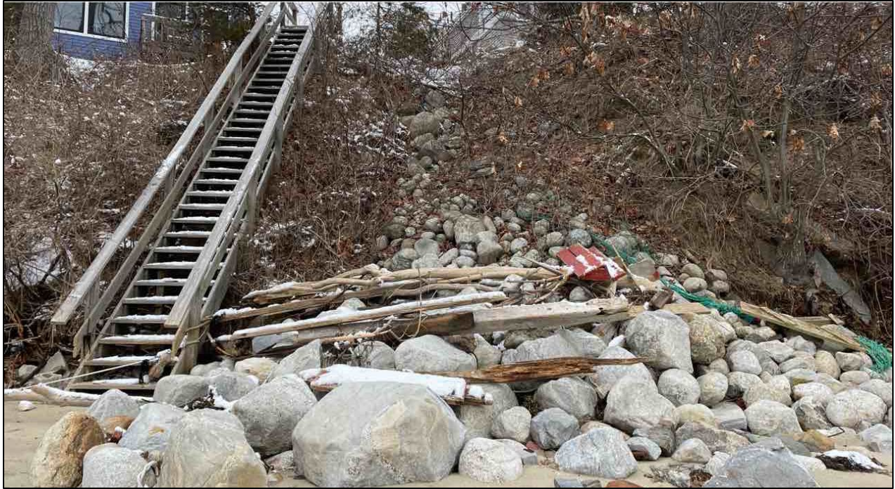
Photograph Three. View of access stairs and the existing rock pile.
