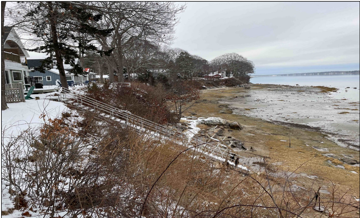
Photograph Four. Additional view of eroding bank from residential structure.
