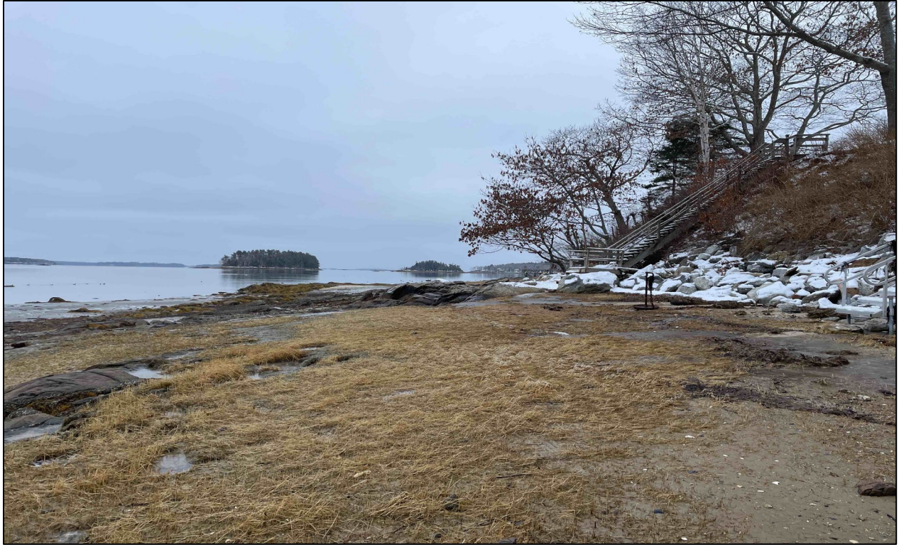
Photograph Three. View of existing access stairs on property. Riprap will continue on far side of stairs.
