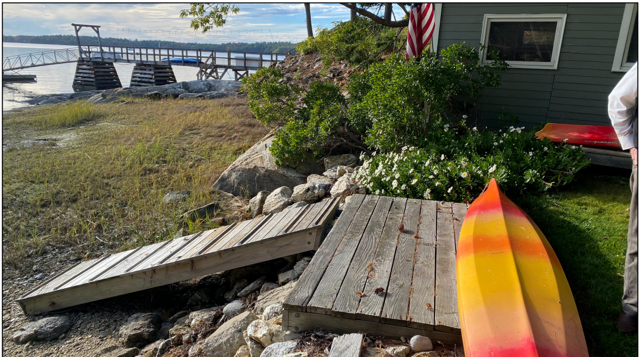
Photograph Four. View of existing ramp and existing wooden landing that is proposed to be replaced with stone. Photographer: Tim Forrester, Atlantic Environmental, LLC. Date: October 4, 2022.
