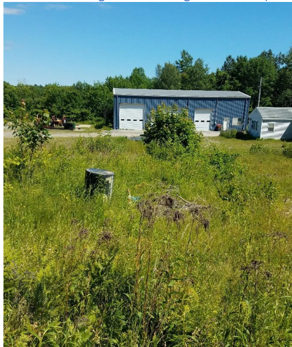
Photo 4. Near western property line looking toward new building location (July 2022, debris has been removed from site)
