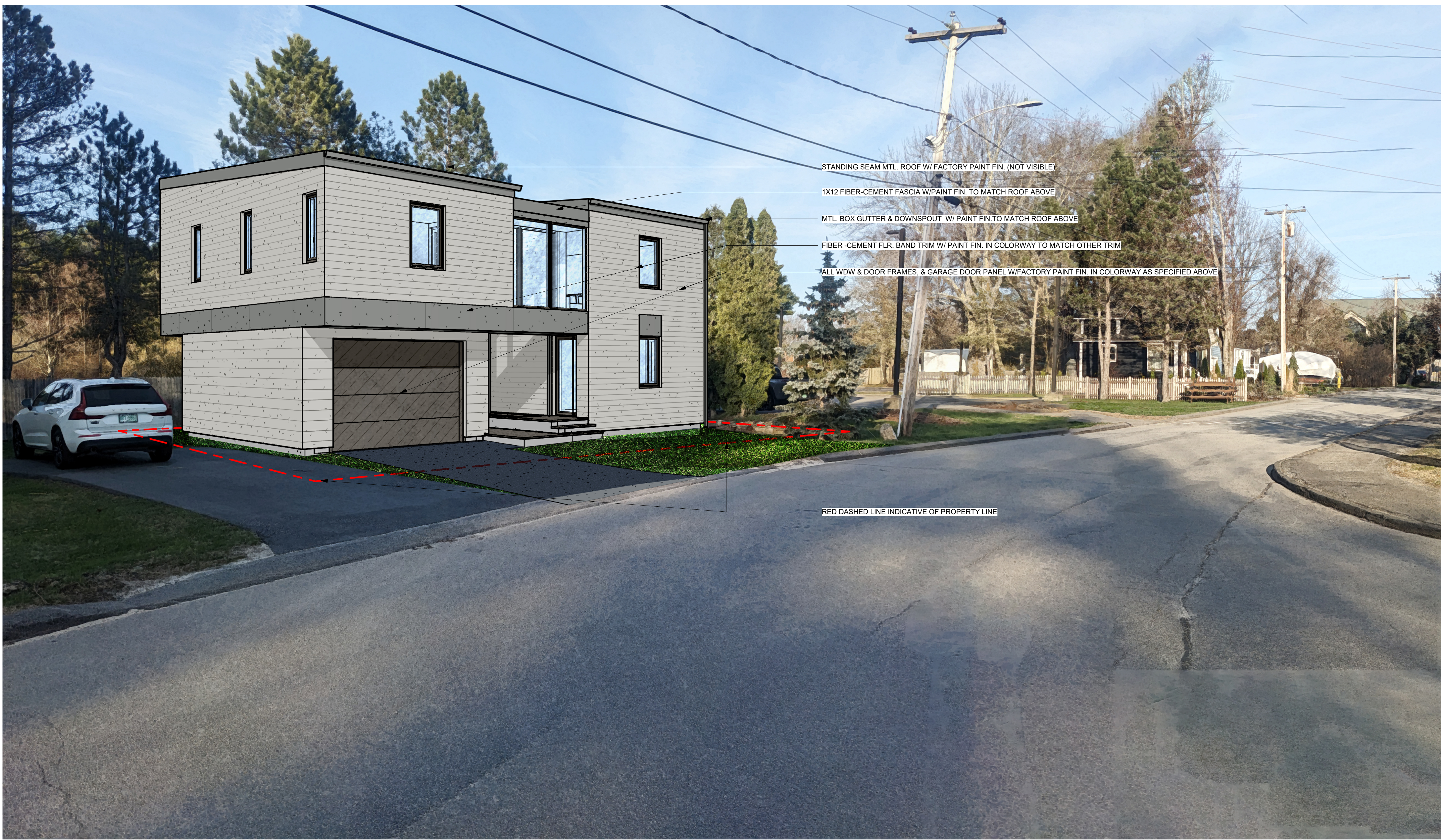
FIBER-CEMENT SIDING JAMES HARDIE ARTISAN SHIPLAP SIDING W/ 9" EXPOSED FACE DIM. IMAGE ABOVE SHOWS SIDING W/ NO PAINT FIN.
